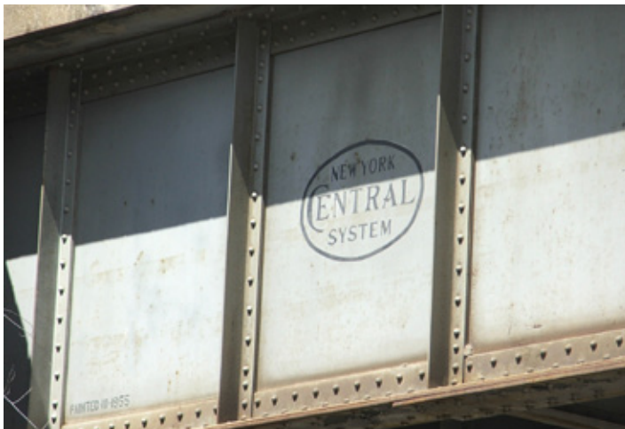
There is no doubt which railroad constructed the River Rd underpass in Little Falls, as part of the mainline relocation project following the tragic Gulf Curve wreck of 1940.
