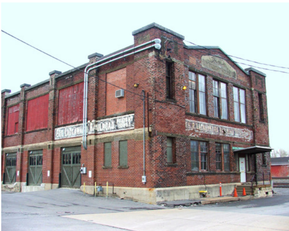
Farther west along the former New York Central (now CSX Transportation) mainline is the Lackawanna Railroad freight house, now used as a yard office and shop by the regional New York, Susquehanna & Western Railway. Both this structure and the old O&W freight house may be easily viewed and photographed from public property along Water Street. Photo by Dave Hamilton.
