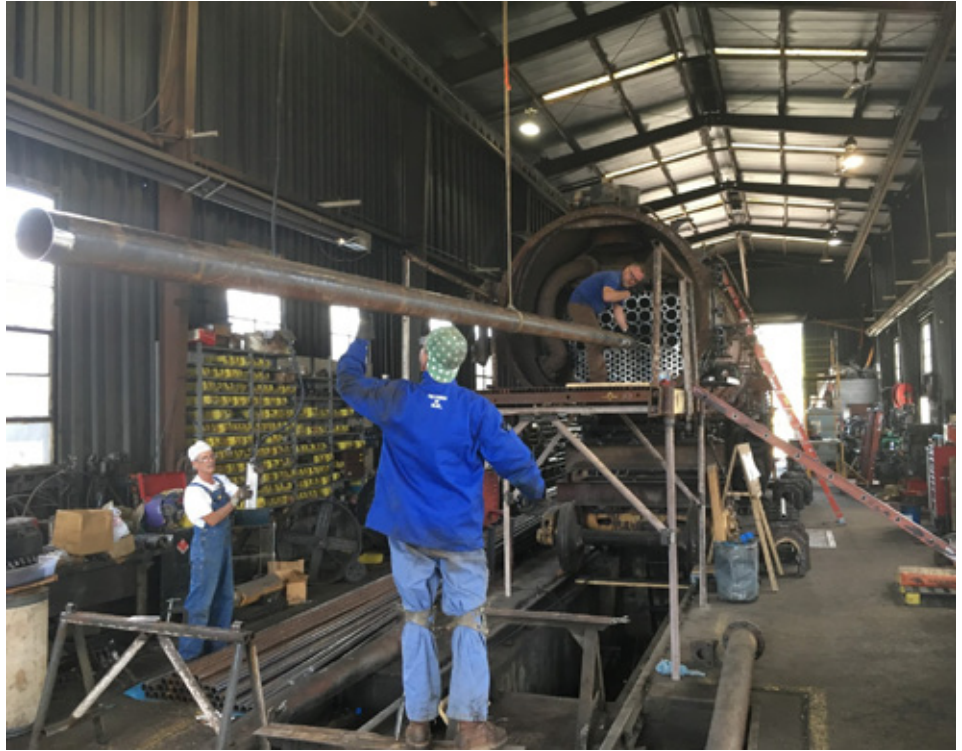
New flues are installed in the boiler of C&O No. 1039, which is undergoing a complete restoration for excursion service. Western Maryland Scenic photo.
