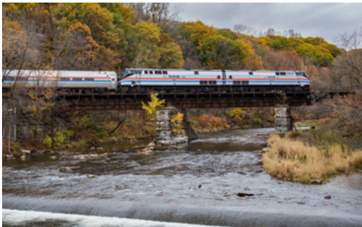
An Amtrak Autumn Express crosses the Hoosac River on the former Boston & Maine Railroad mainline in North Adams, MA. Amtrak photo by Mark Glucksman
