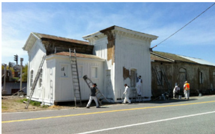
After falling into disrepair over the years, the Rural Retreat, Virginia station has been restored by local volunteers.
