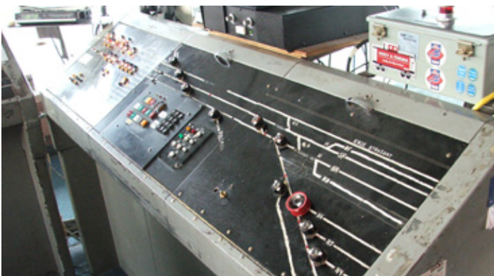
The push-button panel for routing cars in the class yard (above) and the switchtender's control panels (left) were donated to the WNYRHS. Dave Hamilton photos.
