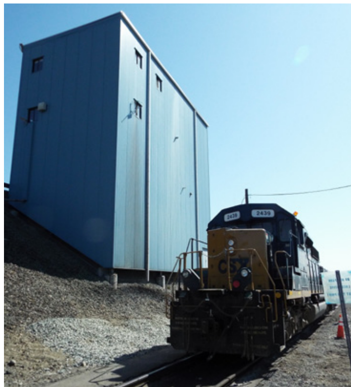
PCRRHS convention tour participants visited the CSX Selkirk Hump tower, opened by Penn Central in 1968.
