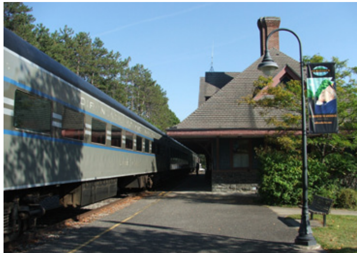
Under a New York State plan to abandon the line, trains will no longer stop at the Saranac Lake Union Station.
