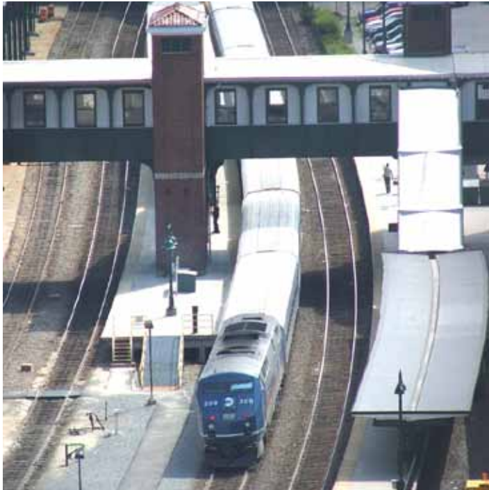
Poughkeepsie station, as viewed from the Walkway.
