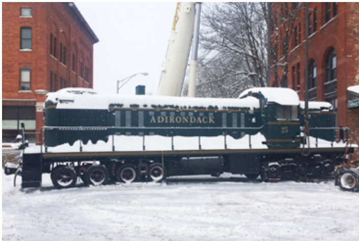
Over the Top Construction crews used a large crane to reposition #25 on rubber tires. John Koslosky photo.
