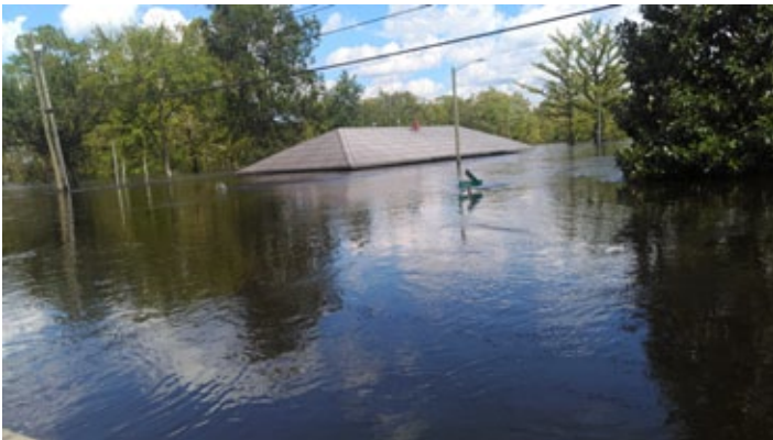
The Pollockville, NC station was totally submerged during Hurricane Florence in 2018. Photo by Mayor Jay Bender.
