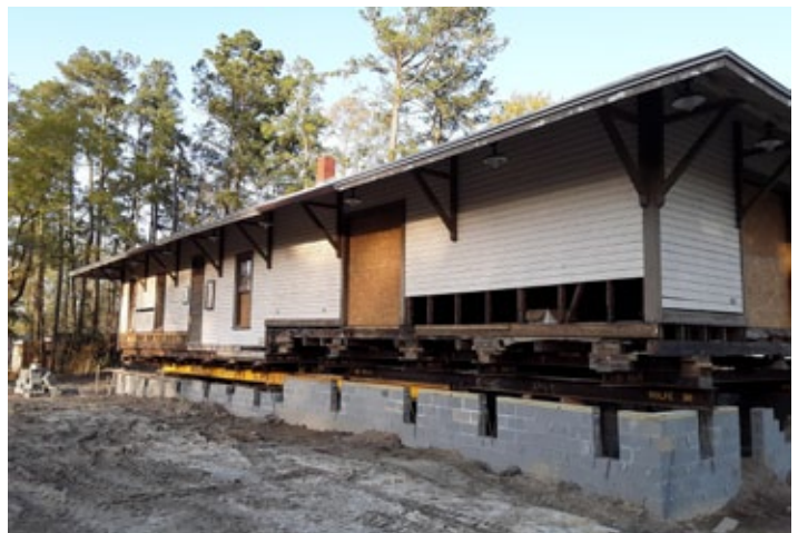
Above, Pollockville station is placed in position at its new location. Below, a new foundation has been constructed and interior work will soon begin. Tom Stranko photos.
