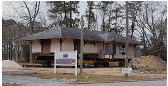
Above, Pollockville station is placed in position at its new location. Below, a new foundation has been constructed and interior work will soon begin. Tom Stranko photos.
