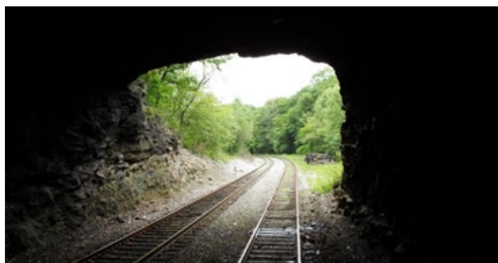
A photo stop at the DL&W Nay Aug Tunnel is planned for this year's Key Lock & Lantern Convention excursion.
