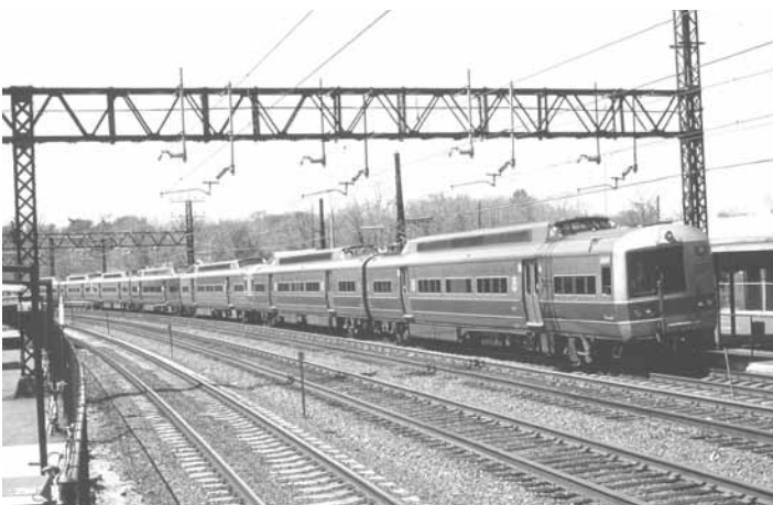
The catenary replacement project on the New Haven was complete when this photo at Rye, NY was taken in 2003.
