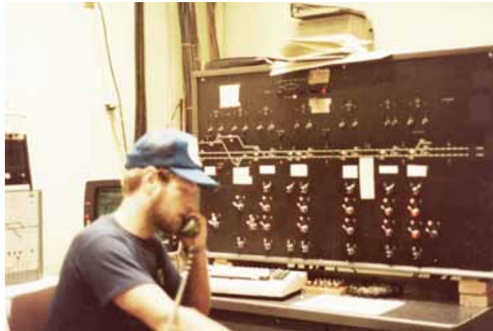
The St. Lawrence Desk, which controlled the "dark" territory from Syracuse to Montreal, was given charge of the Hudson Line from Albany to Poughkeepsie in 1983. Dispatcher Mark Gravelin lines up an Amtrak train on the board in this 1984 photo from the collection of Bill Moll.
